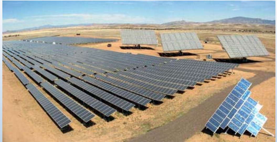
PV systems at the Arizona Public Service facility in Prescott, Arizona
