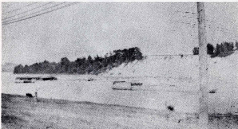
A part of the old Veazie Dam
