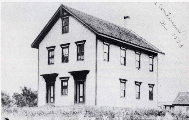
The High School-Grade School Building
