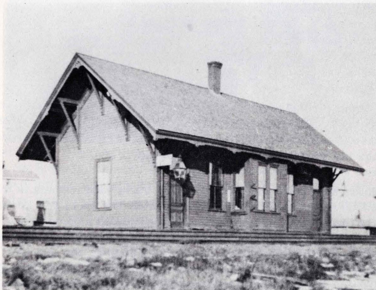
Train station located on School Street
